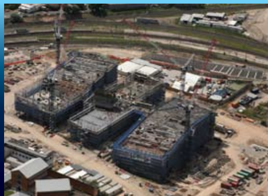
Construction of the Boggo Road Ecosciences Precinct progresses
